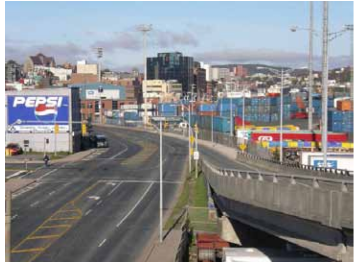
Looking east along the route of the harbour inteceptor sewer - a trench 7 x 7 m will be dug along the south margin of the roadway. (G. Penney)
